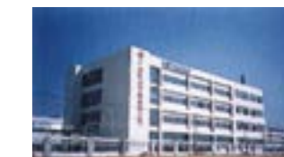
Hitachi Air Conditioning & Refrigerating, Китай
